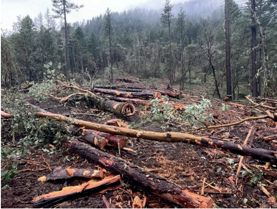
Extensive hardwood removal in unit 5-6 of the Apple Saws Timber Sale. The photo shows whole slopes cleared of both live conifers and live hardwood trees, including black oak and Pacific madrone. Photo taken by Luke Ruediger on February 8, 2026. See Decl. Ruediger, Fig. 4.
