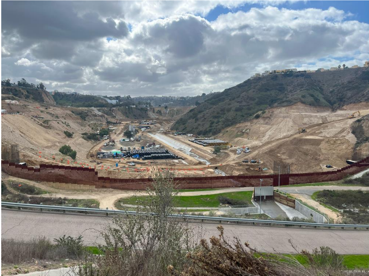
Figure 13: Mexican Construction Project in Matadero Canyon. (MC 01/10/2024)
