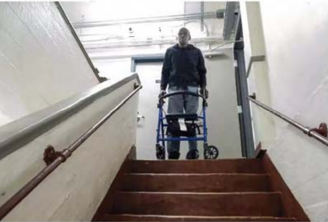
Kenneth Owens, 70, stands at the steps with his walker inside the Madison Hotel, which is owned by the AIDS Healthcare Foundation. Owens is one of 18 tenants who sued the foundation over a chronically broken elevator. (Francine Orr / Los Angeles Times)
