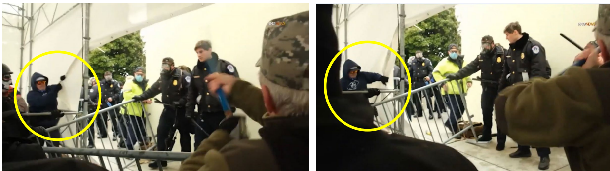
Ex. 423 showing Bozell (yellow circle) tearing the tarp under the scaffolding
