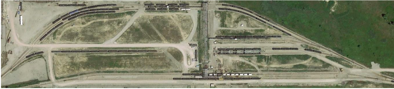
Figure 28: Imperial Nanticoke, ON Rail Infrastructure 79
