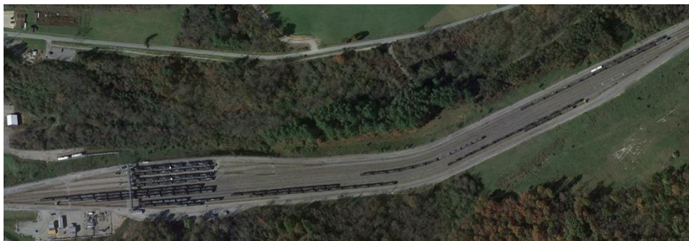
Figure 71: Blue Racer – Proctor, WV Rail Infrastructure 161
