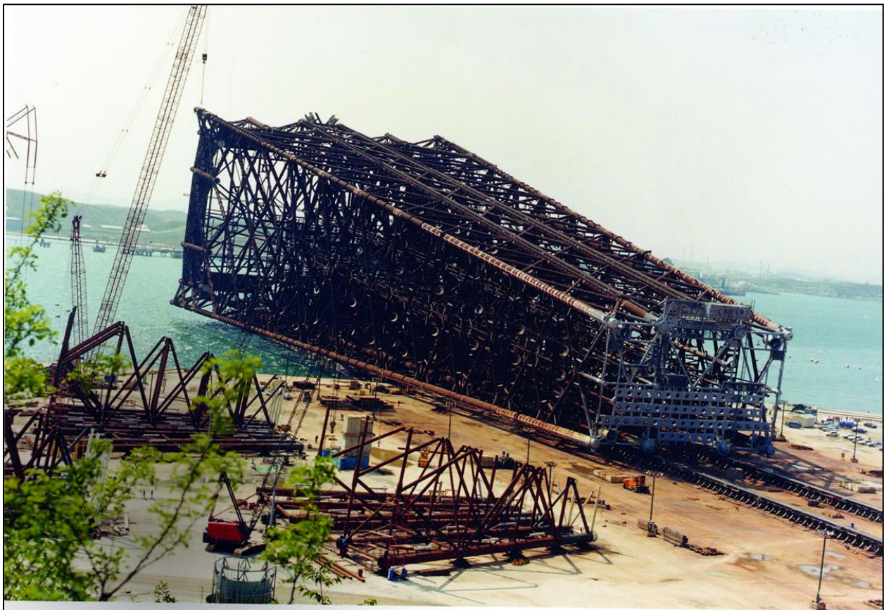
Figure 8. Platform Harmony jacket onshore prior to installation (Bull 2018)
