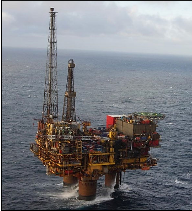
Figure 13. Photo of Brent Delta prior to decommissioning in the North Sea (Adams 2015)
