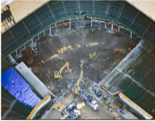
During construction behind home plate
