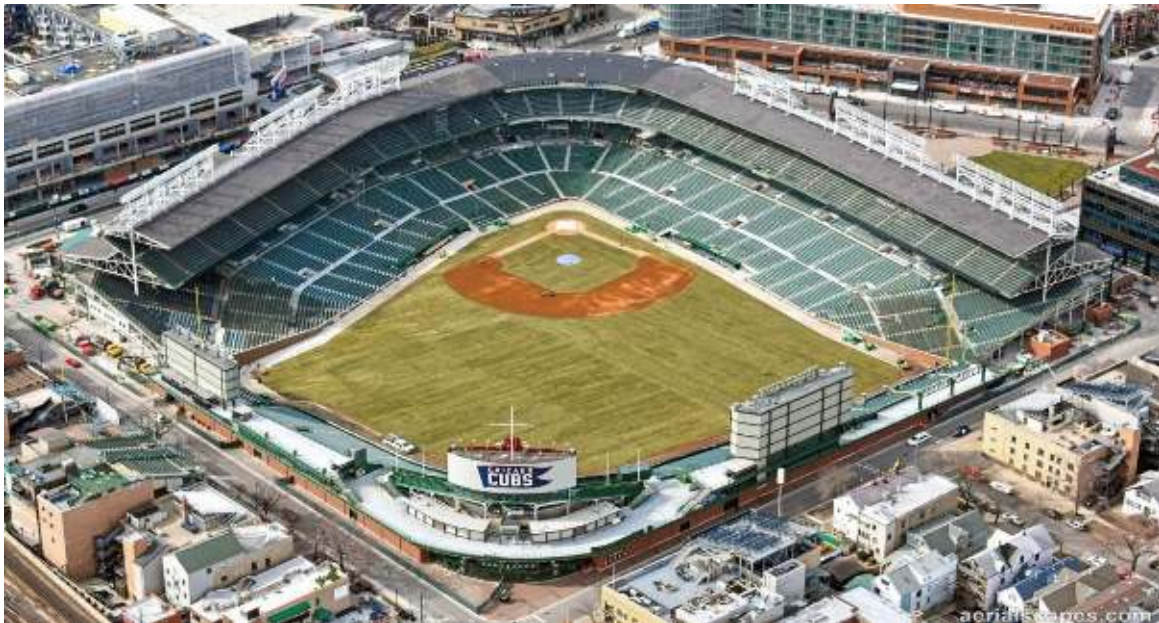
Lower grandstand after construction
