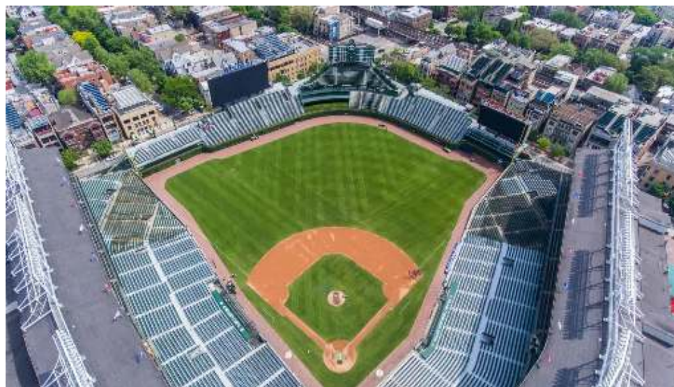
Outfield bleachers after construction
