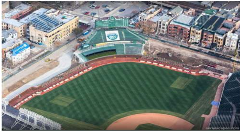
Outfield bleachers during construction
