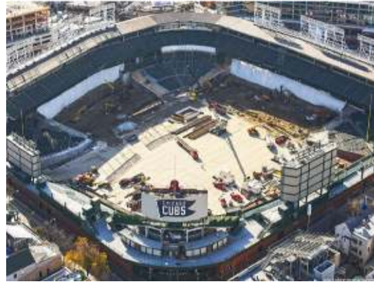
During construction down first and third base lines
