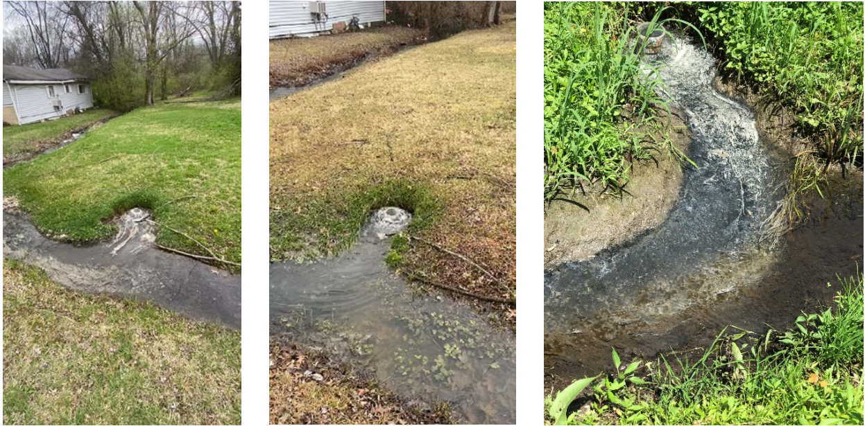
Figures 10-12: Dry weather sanitary sewer overflow at North 82 nd Street in Centreville, Illinois on March 30, 2021, January 26, 2021, and June 26, 2019, respectively, from left to right.
