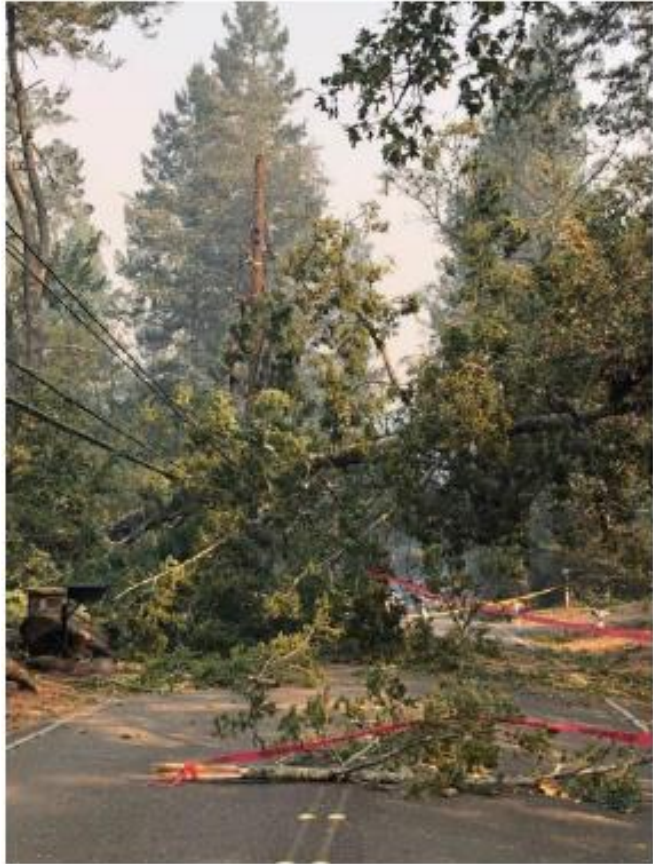
A blown-over tree and broken conductors in Sonoma County.
