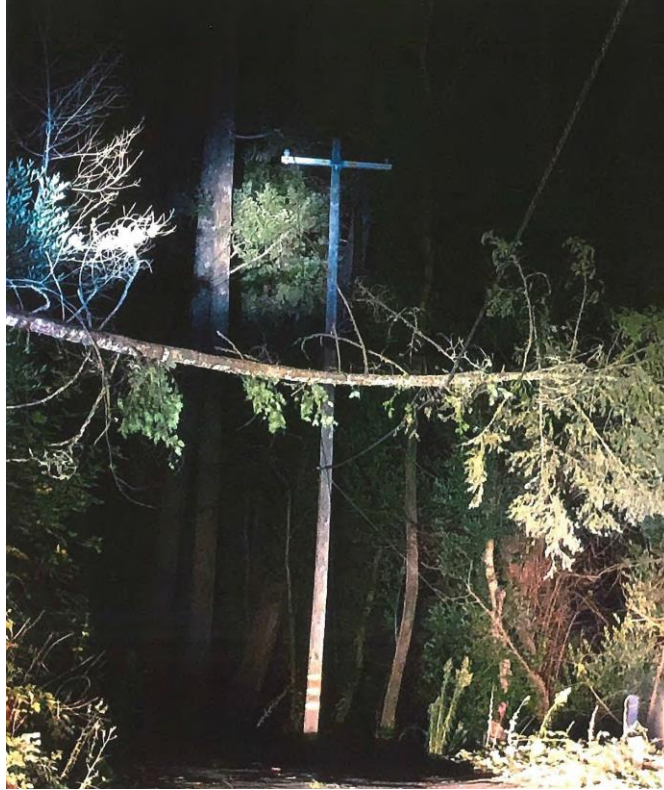
A tree blown onto conductors in unincorporated Napa County.
