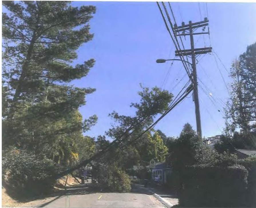
A tree blown onto conductors in Alameda County.
