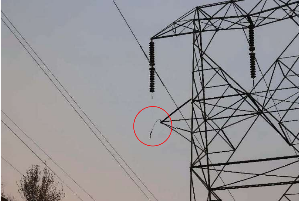
Figure 2. At Tower :27/221, an insulator hold-down anchor was disconnected. Photo provided by PG&E. 78
