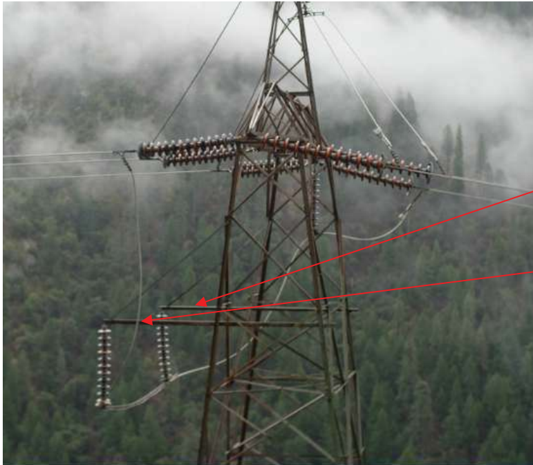
Figure 8. Typical location of runner arms on transmission towers similar to the Incident Tower. This is PG&E Tower :20/160 of the Caribou-Palermo 115 kV Transmission Line. 84
