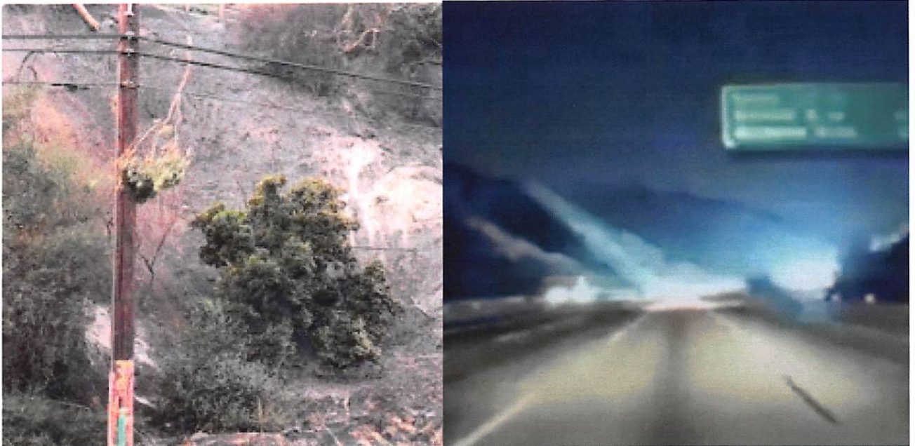
7 8 9 10 11 12 13 14 15 16 17 Remains of the branch that struck LADWP's sub-transmission lines (left), and a freeze-frame of the dash-cam footage 18 that captured the electrical event. ( https://www.lafd.org/news/getty-fire , November 19, 2019)
